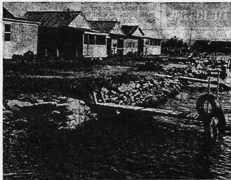
Some of the threatened houses on Coon Island.
