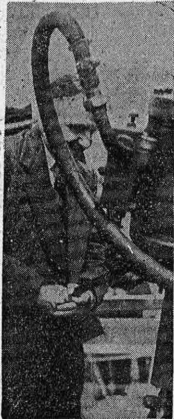
Mr. G. Booth, M.L.A., drives the first rivet in the keel of a freighter to be built at the State Dockyard.
