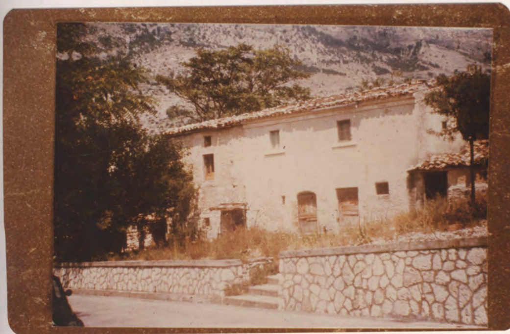
Plate 9: Stables Converted to Homes, Now Derelict
